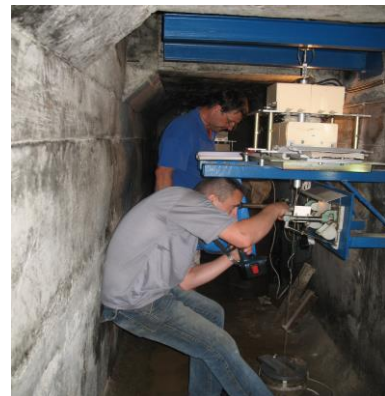
Installing the DAQ system inside the dam
